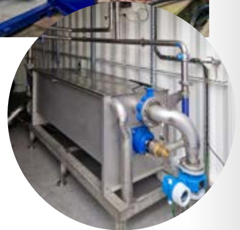
Compact and efficient integration of the wastewater heat exchanger within a retrofitted container.
