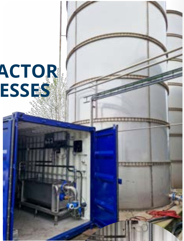
Compact and efficient integration of the wastewater heat exchanger within a retrofitted container.
