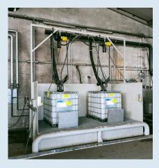
temperature, pH and the degree of pollution are continuously monitored. If necessary these parameters are automatically adjusted to the desired level.
